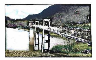
Nuuanu Reservoir No. 4 features a tower which contains three gates or valves which help regulate the water level.
